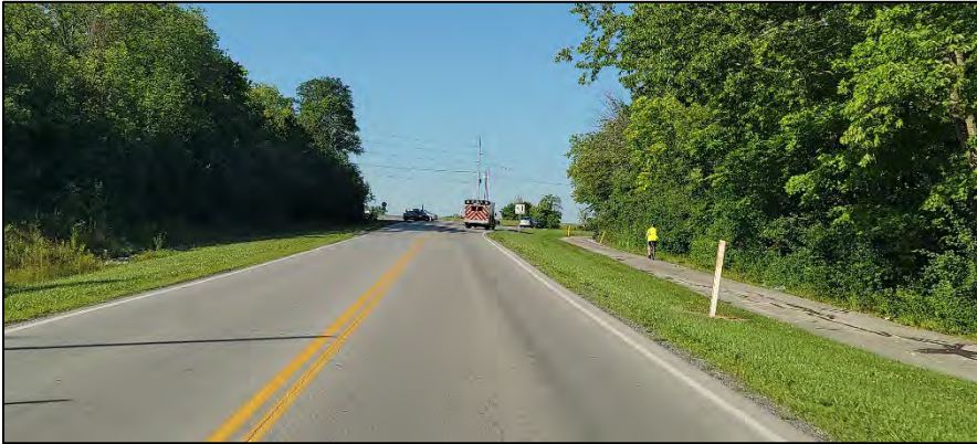
Photo 1: Adjacent shared use path located along west side of Ft. Amanda Road along the Ottawa River
